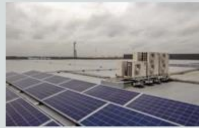
Picture 1 (left): Charging area in the warehouse, subject to temperature control Picture 2 (above): Roof of the office space equipped with the LG air to water heat pump and LG PV panels Source: LG
