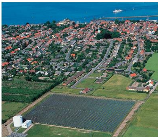
Marstal/ Denmark, 18.300 m 2 collectors, 10.000m 3 buffer storage, 30% of the local heat delivered, Energy woods need > 10 times larger land area!
