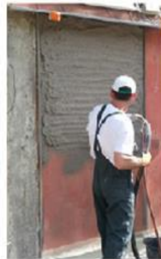
Silica aerogel based thermal mortar – methods of façade wall application
