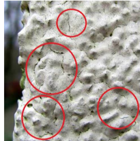
Deformations of different facades a) facade coated with conventional paint; b) facade coated with nanocoating
