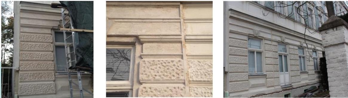
Renovation of a historical building façade with aerogel thermal plaster
