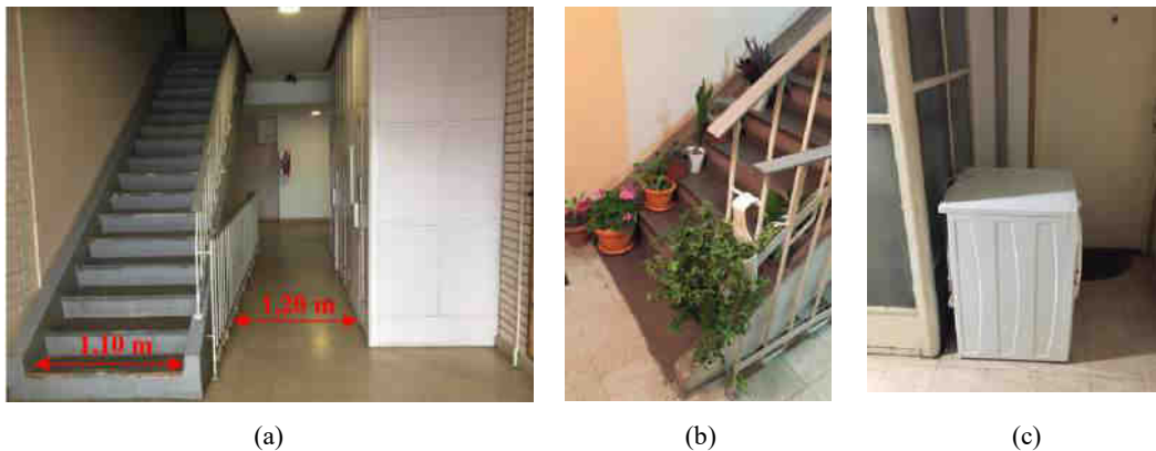
Figure 8 – Evacuation routes: (a) insufficient width of the main staircase and hallways; (b) obstacles in the form of potted plants; (c) obstacles in the form of furniture;
