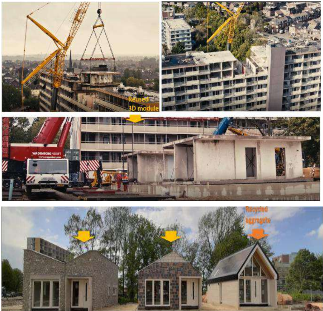
Figure 7- Hoisting of elements and two 3D units for the construction of two circular houses (Type A left and Type B middle). The structure for the third house (Type C) has been made of recycled concrete.
