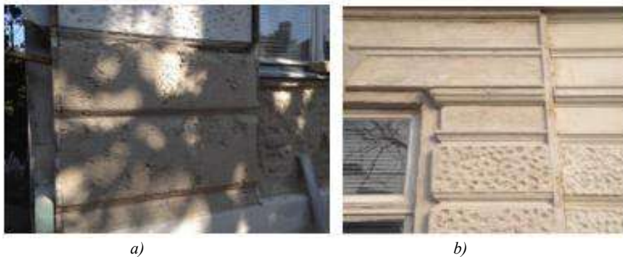
Figure 3 - Old renaissance building façade, a) original material before aerogel plaster application; b) after aerogel plaster application
